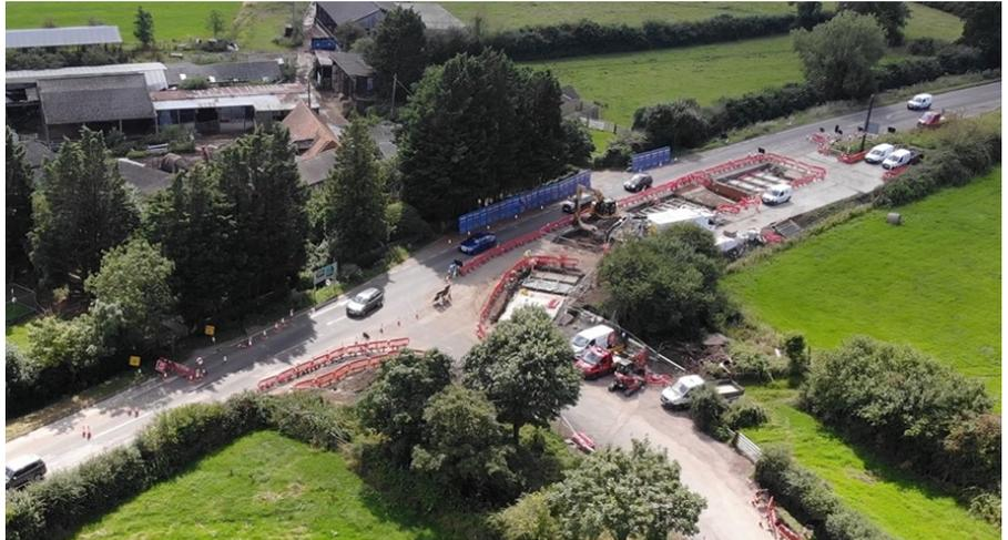
The Project required the complete reconstruction of 1.5 km of the existing Station Road carriageway and also to complete improvements to the existing priority junction of the A41 and Station Road, in order to cater for the increased traffic flows associated with HS2 construction work. The A41 carries traffic from Bicester to Aylesbury and Station Road serves the village of Quanton, with the access to the HS2 works site compound circa 1700m along Station Road.
